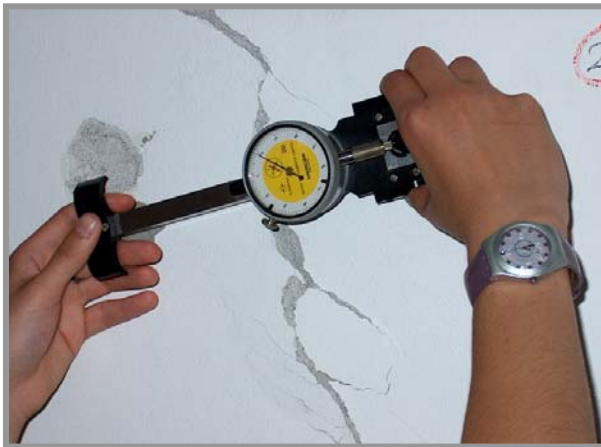
FIG. 5 – DEFORMOMETRO IN OPERA
